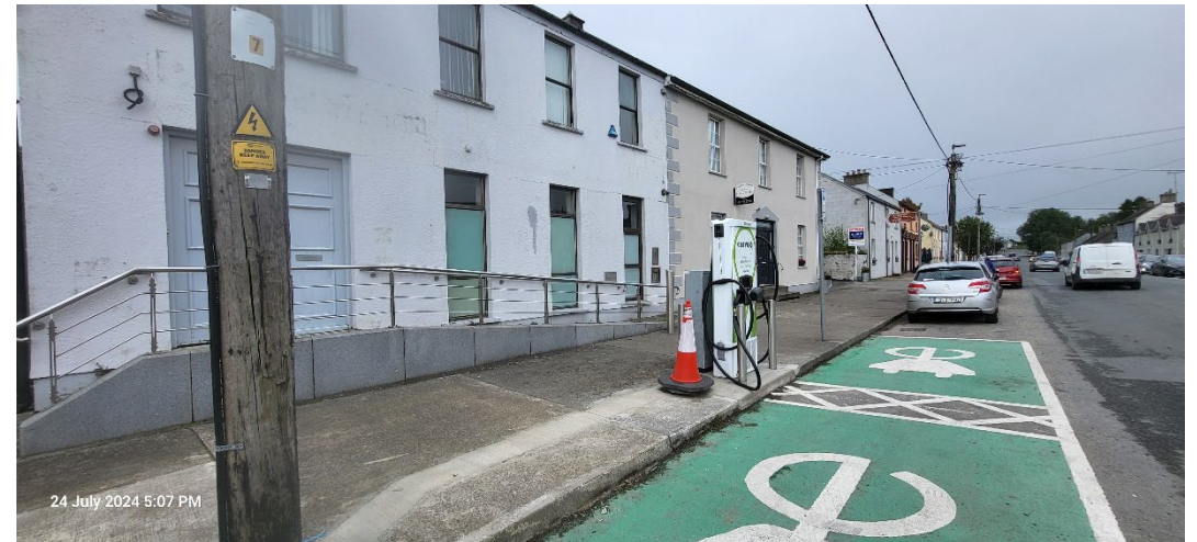
Front entrance ramp and Car Charging Area
